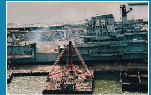
PIER BREAKING / ALONGSIDE
